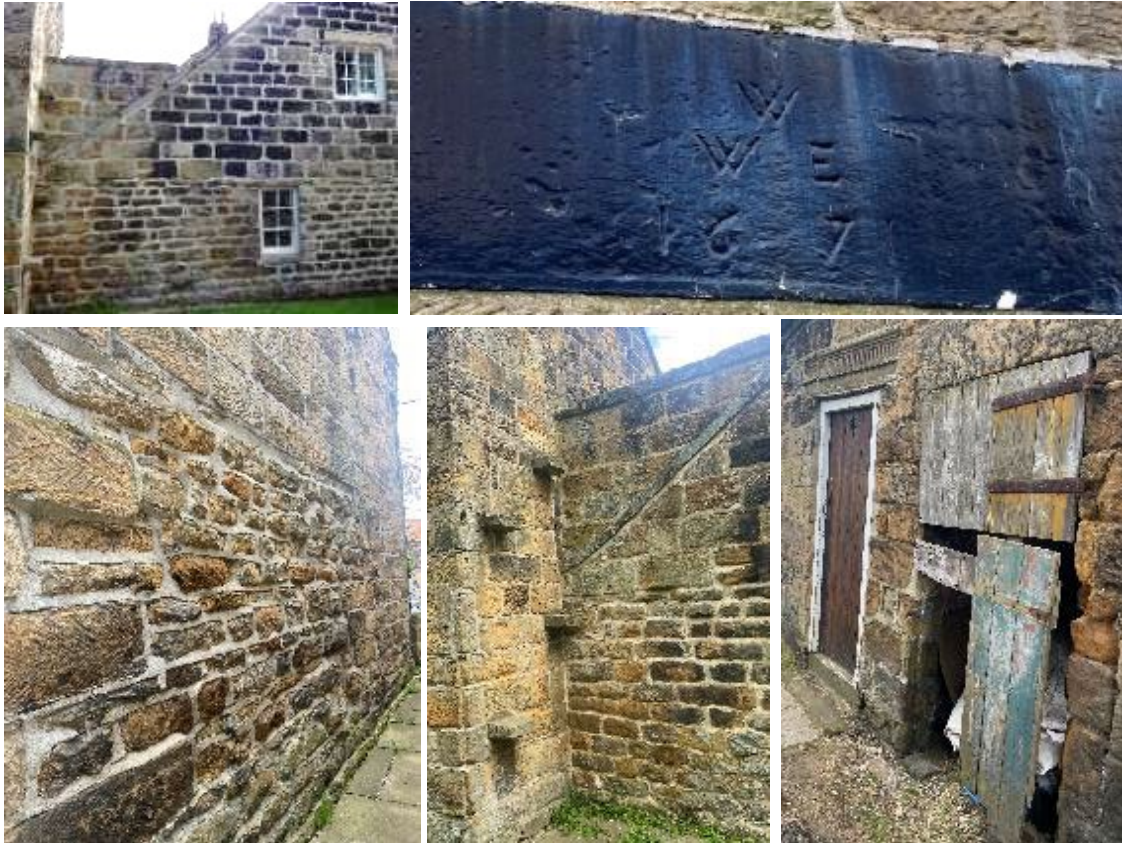
Figures 09-13: Images of scarring, previous openings, mason's marks and varied building materials. Materials may have been re-used from the castle, with variations in stone tooling.
