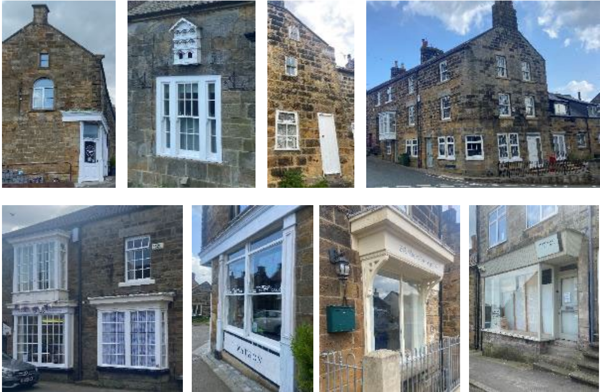
Figures 71-82: A range of traditional windows and shopfronts in Castleton. A clear hierarchy of windows from ground to upper floor and a mix of modest and ornate styles and detailing.
