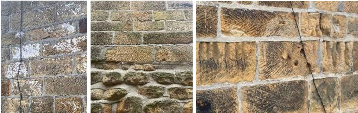
Figures 53-55: A variety of tooling styles and possibility of surface finishes.
