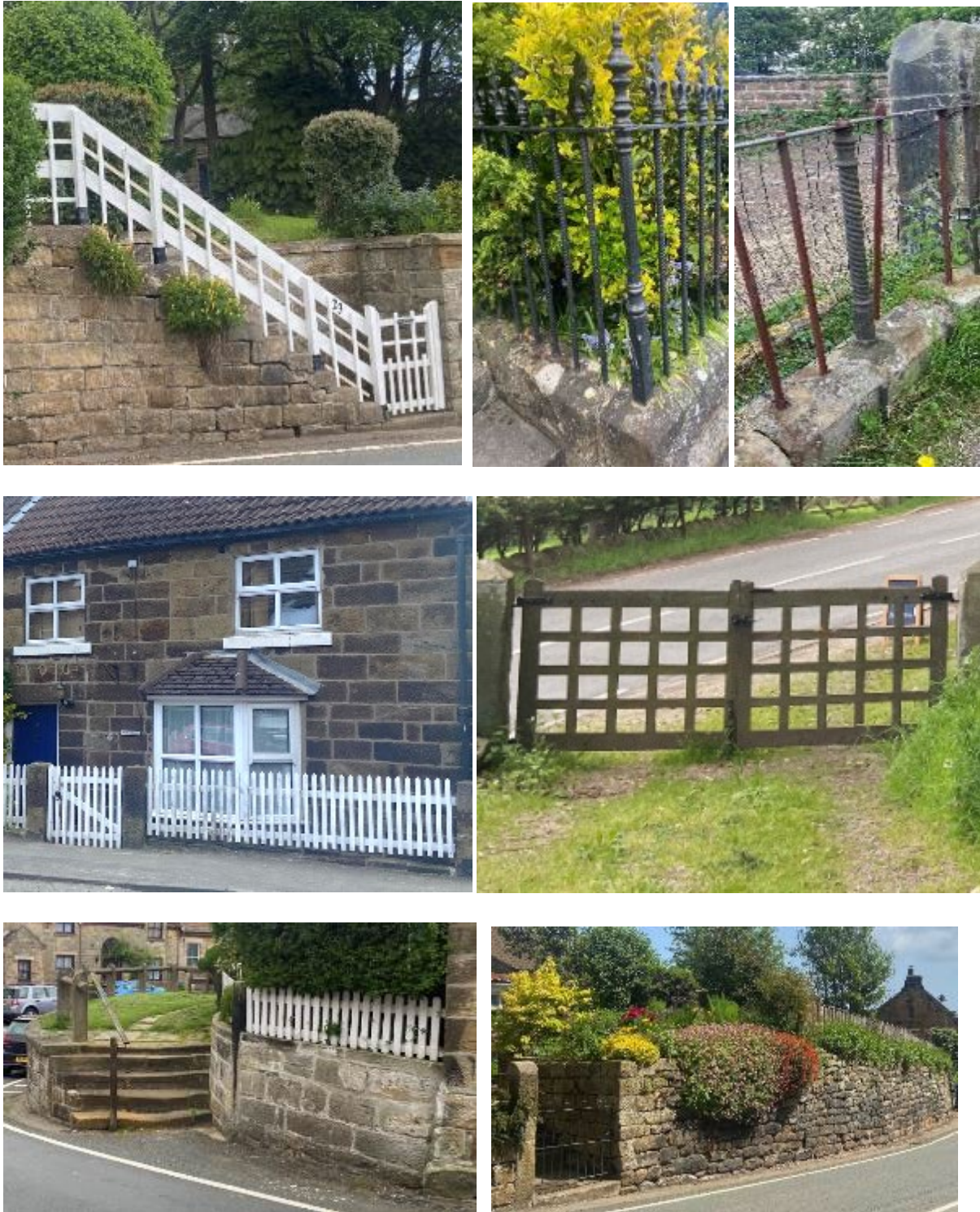
Figure 32-38: A variety of boundaries in Castleton, including stone, timber fences, stone steps, iron railings and gates.
