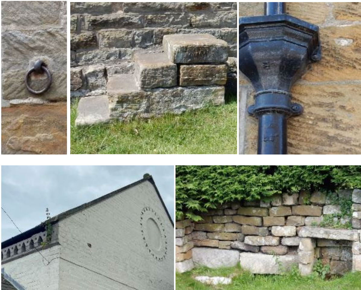
Figures 83-87: Small and often hidden details that positively contribute to the character of the area. Some included here are horse ties, stone mounting blocks, building details and cast-iron painted rainwater goods.
