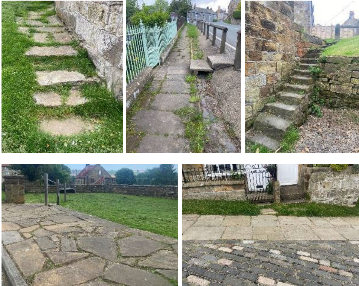
Figure 23-27: Examples of surface treatments including paving, steps, cobbles and trods.
