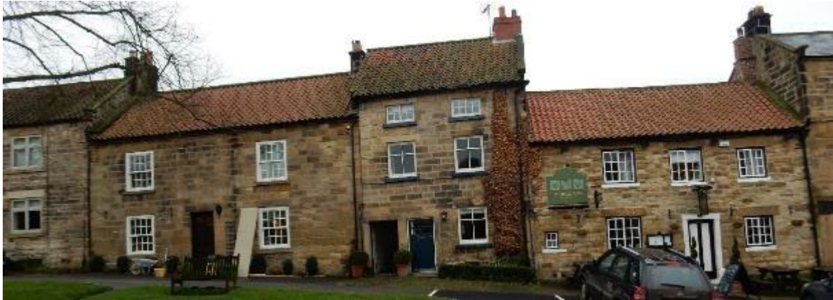
Figure 38: A row of mainly Georgian frontages on South End with a mixture of roof heights which is distinctive to the village and window types representing the traditional Yorkshire sliding sash, 8/8 sliding sashes and modern replacements. The tall central building retains a cross passage next to the house door.
