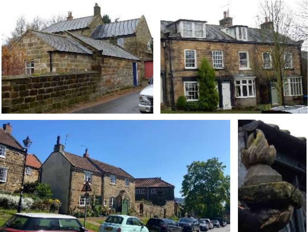
Figures 51-55: A range of roofing details, featuring slate and pantile at a variety of orientations.
